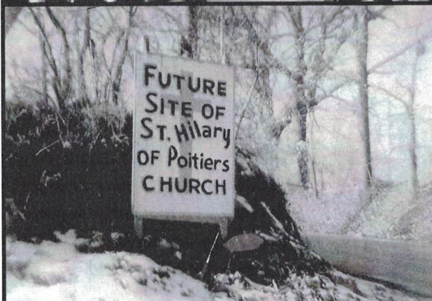
Site of the Parish Plant before Groundbreaking
